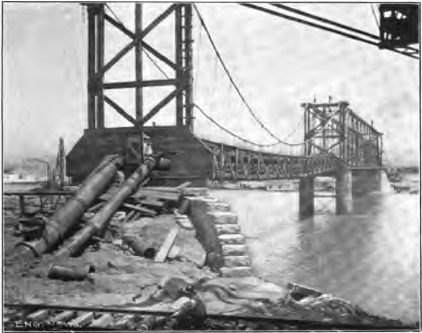
FIG. 2. SUSPENSION SPAN OF FLOW-LINE BRIDGE.
